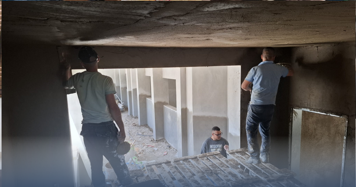
Construction site of the Palestine School in Dura.
